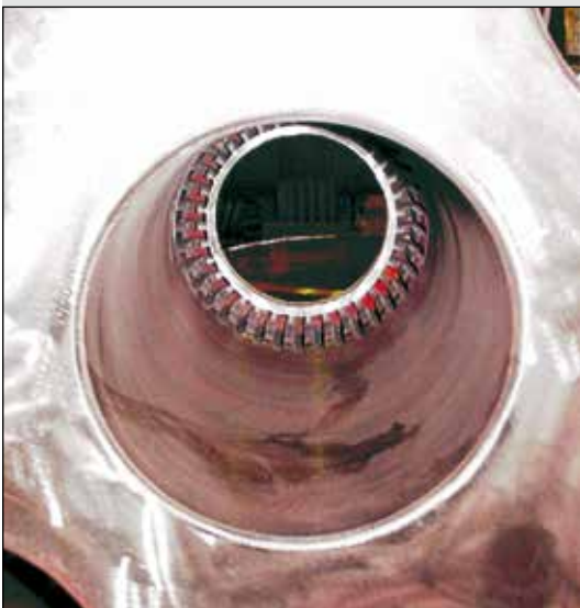
Reinforcement ribs on waterside of the gas inlet nozzles
