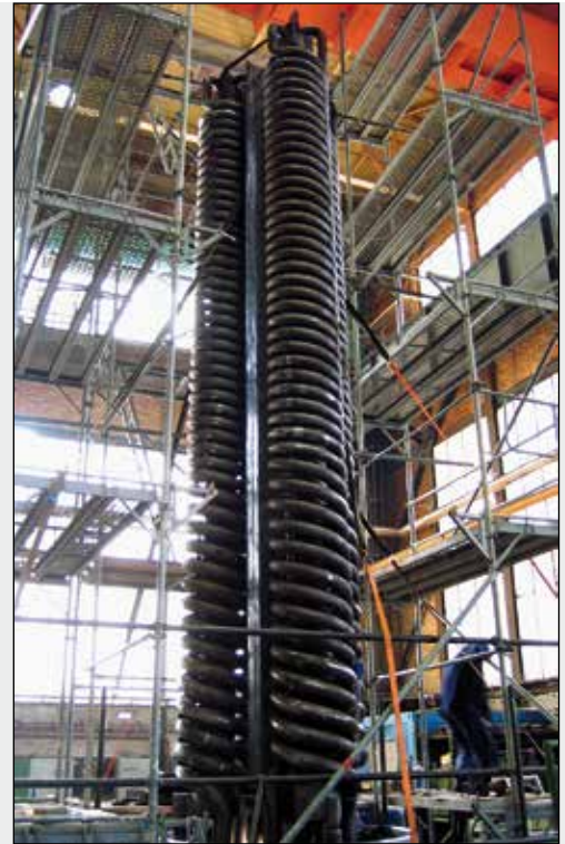
Assembly of coils
