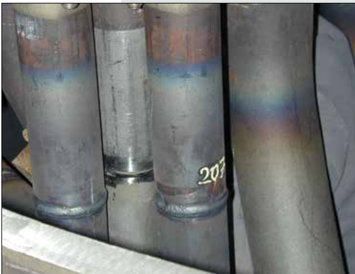
Fitting and welding of heating surfaces to connecting tubes
