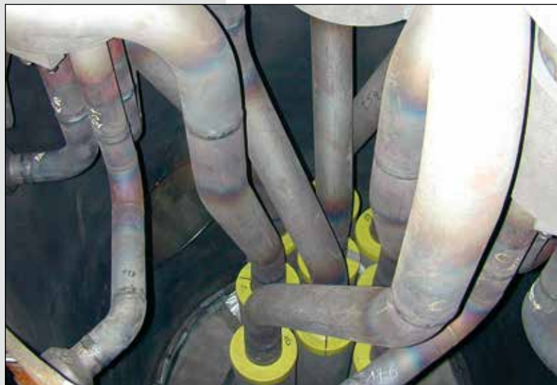
Assembled tubing between heating surfaces and inlet section
