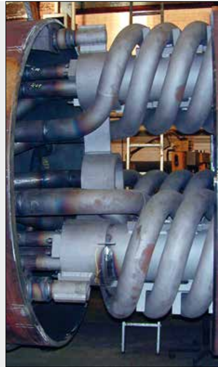
Final assembly of boiler shell
